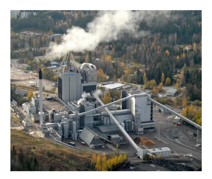
constructed. The automation keeps the electricity and heat generation constant with about 200 guided motors, almost 1,000 measuring points and a price tag of nearly €10 million. In addition to SRF, the plant uses some actual natural gas, e.g., to start up the gasifier, and ignite the burners of the boiler as well as during situations when the plant malfunctions.
